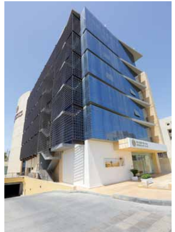
The entrance to the Shmeisani branch at INVESTBANK's head office building
