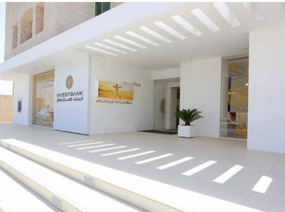
The contemporary façade of the Abdoun branch complete with INVESTBANK's signature logo and sun-saturated imagery
